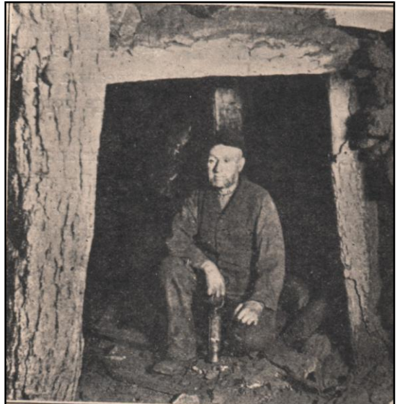
Miner in a manhole underground
