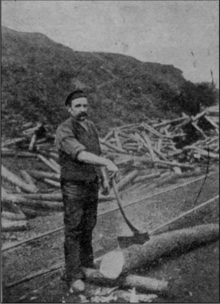
A timberman cutting arms and collars
